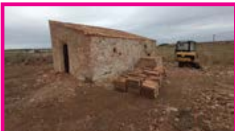
Building work in progress
