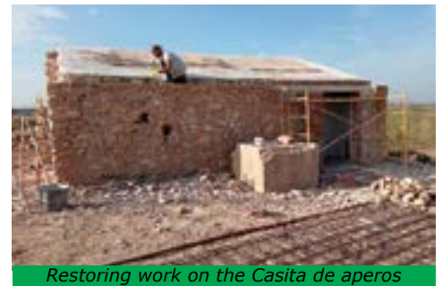
Restoring work on the Casita de aperos at the ranch
